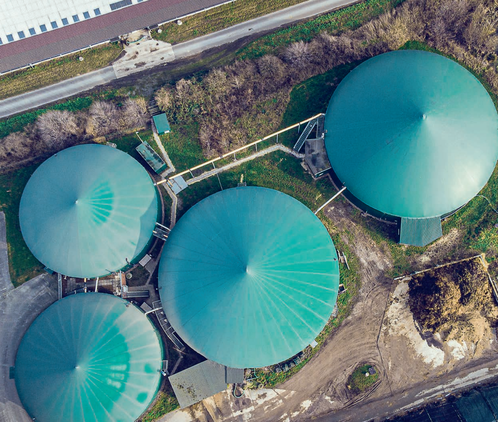
Biogas plant in Osterholz-Scharmbeck, Germany
